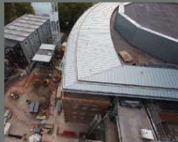
The new roof that oversails the restaurant has been completed.
